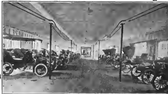
Interior view of Auto Garage.
